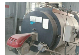
■ Air supply fan for boiler
