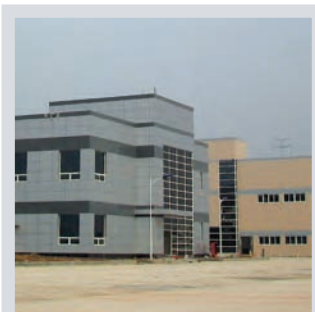
Wuxi Plant (China)
